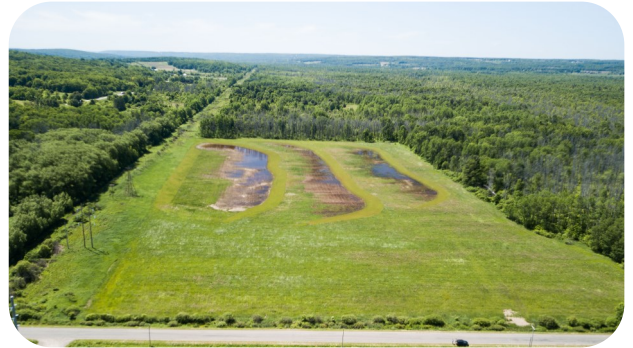
A drone photo showing recently constructed wetlands created by Ducks Unlimited on the site.
