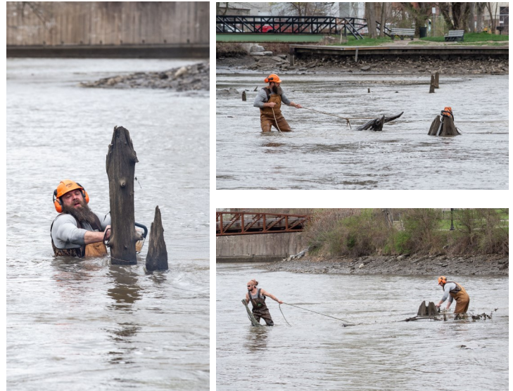
Tactical Tree Solutions removed tree stumps and vertical spikes from the Chadakoin River basin for safer navigation.
