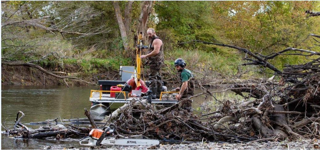
Barge-mounted crane in use – on-water hazard removal – Upper Conewango Creek, Kennedy, NY.
